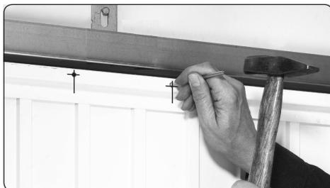
2. Punch in the fixing holes in the door frame with the aid of the enclosed spike
